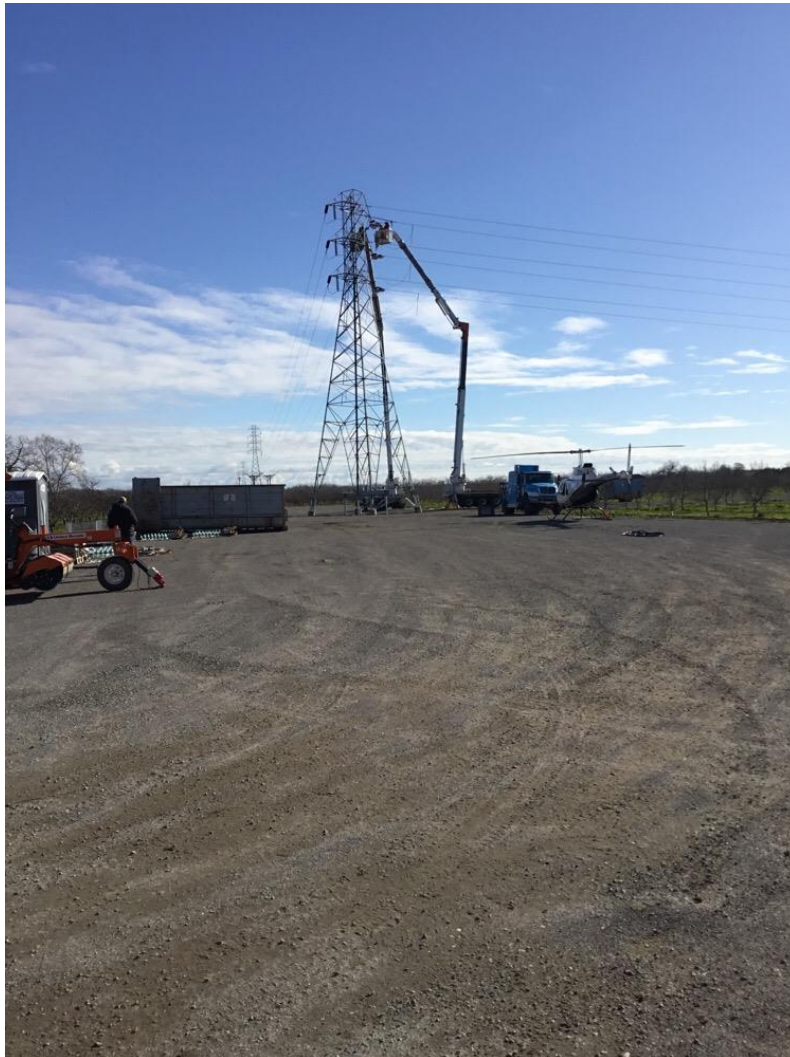
Photo 2: Crews installing rollers at structure 4/24.
